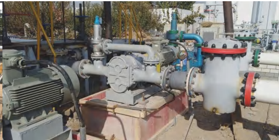
Lobe Pump (with Basket Filter and Safety Valve) Application to Chemical Industry
