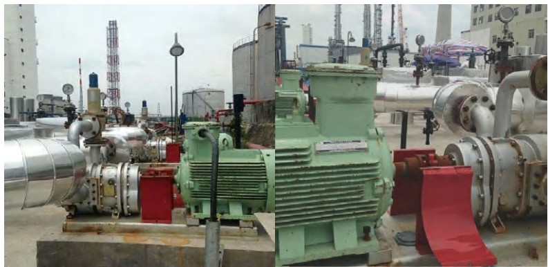
Lobe Pump for Asphalt Transfer
