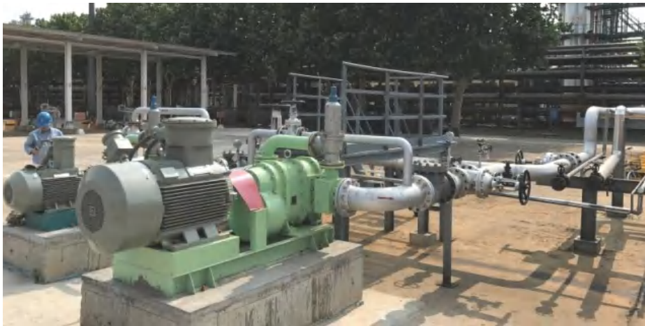
Lobe Pump (with Basket Filter and Safety Valve) Application to Chemical Industry
