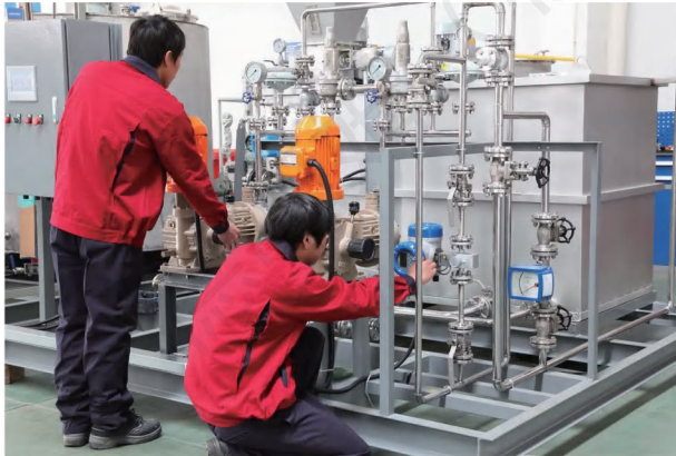
Meticulous Material Reinspection
