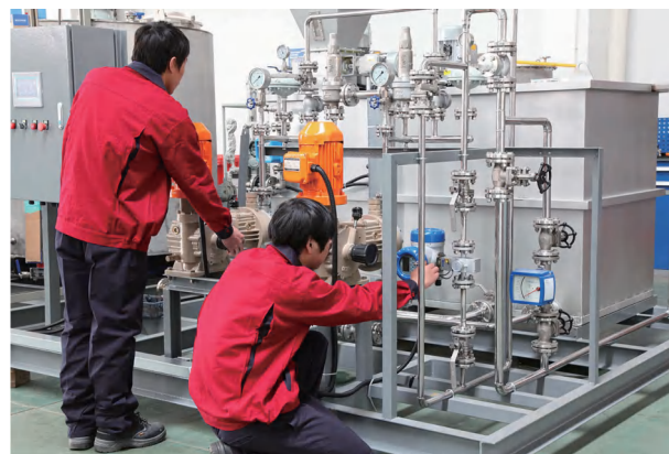
▼ 精心材料复验 Careful Material Reinspection
