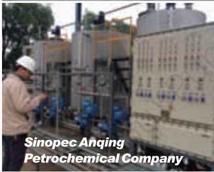
Sulfuric Acid (H 2 SO 4 ), Sodium Hypochlorite (NaClO) and Stabilizer Injection System
